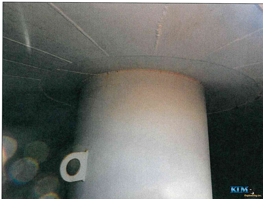
Photo No. 6 Top of the drywell tube
