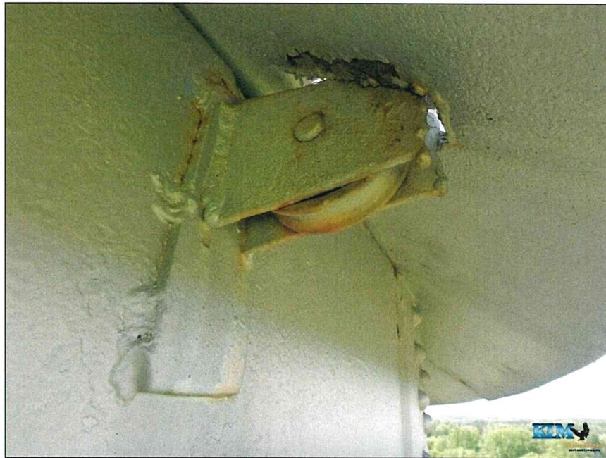
Photo No. 23 No longer used water level indicator rope sheave
