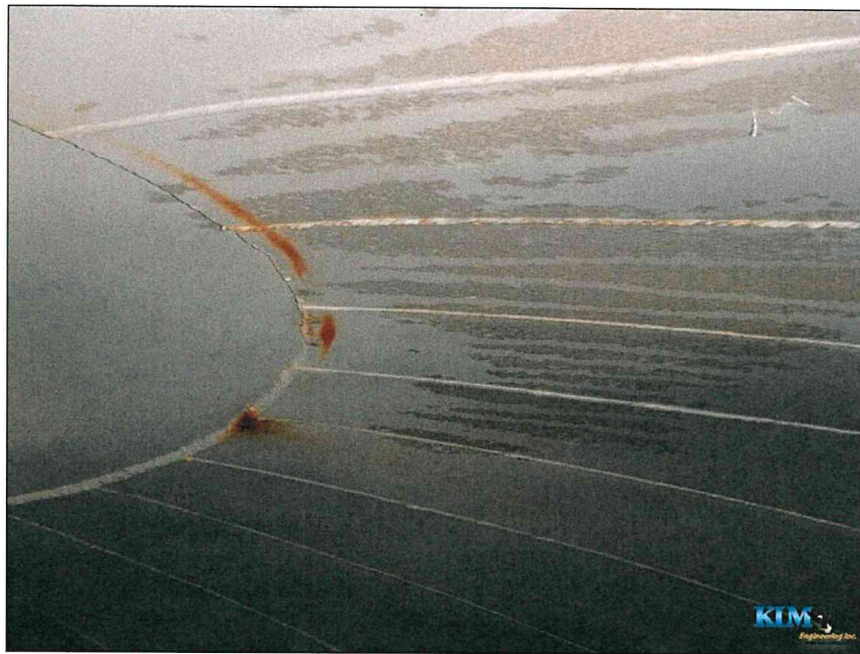
Photo No. 3 Condition of the roof plates
