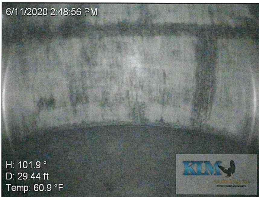
Photo No.16 Condition of the floor and bottom shell course
