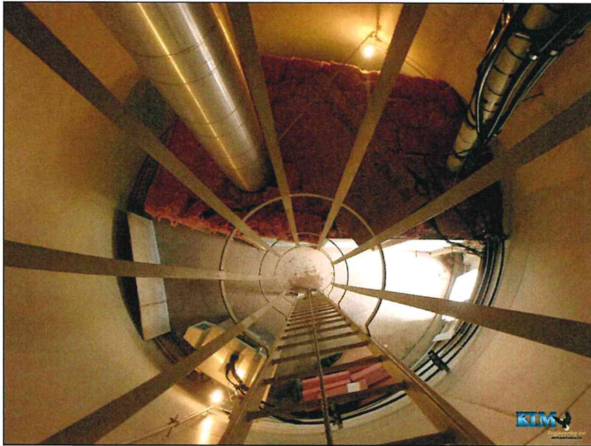
Photo No. 31 Overall view and condition of the base cone
