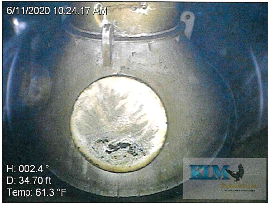
Photo No. 19 Bowl inner cone access manway
