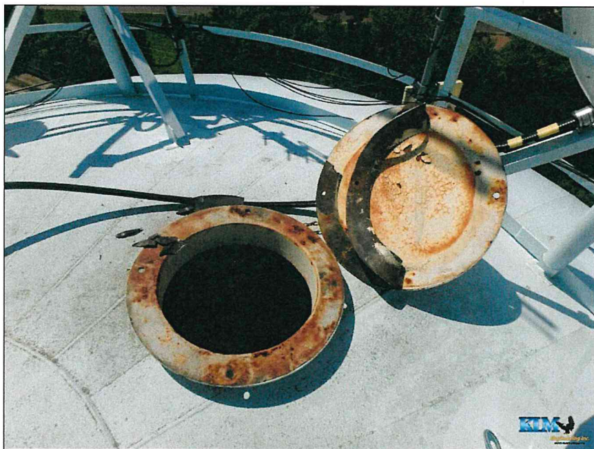
Photo No. 36 Condition of the ventilation manway
