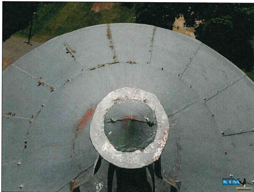
Photo No. 18 Condition of the roof
