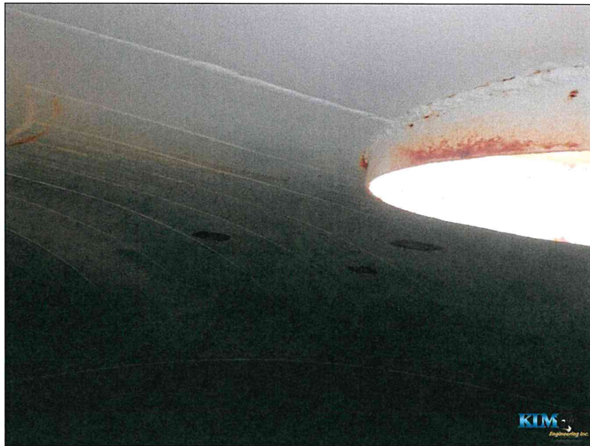
Photo No. 7 Condition of an access opening curb
