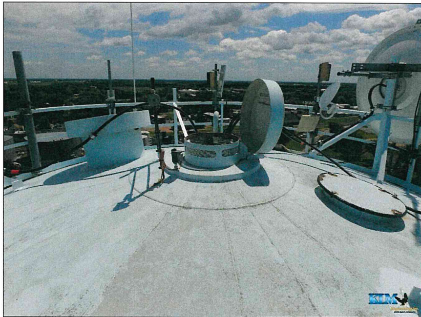
Photo No. 35 Overall condition of the roof
