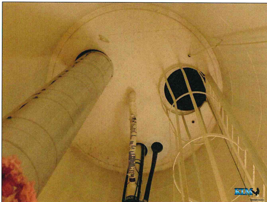
Photo No. 30 Condition of the underside of the lower landing
