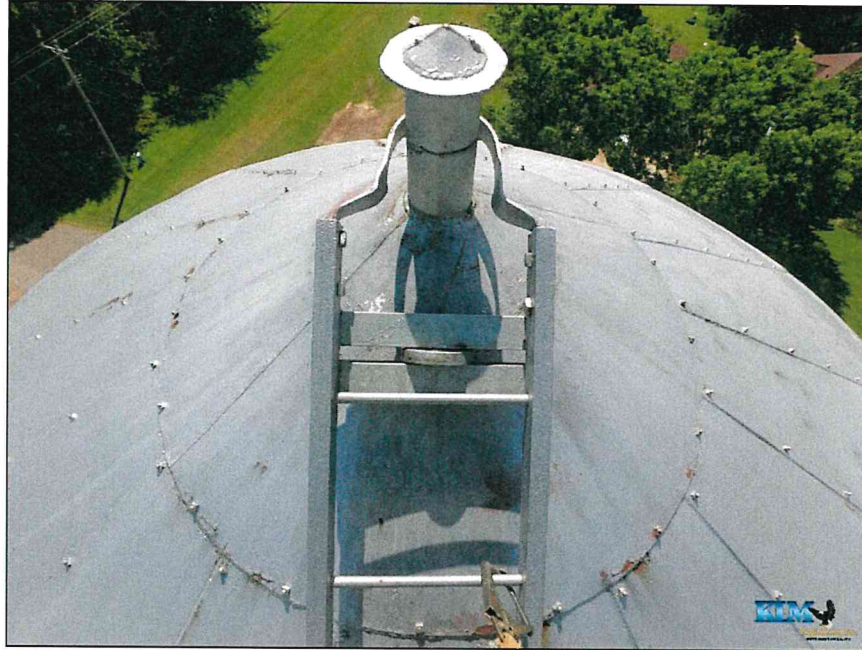
Photo No. 17 Overall condition of the roof
