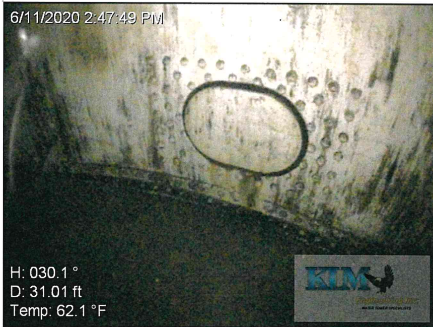
Photo No. 13 Condition of the base shell course with access manway
