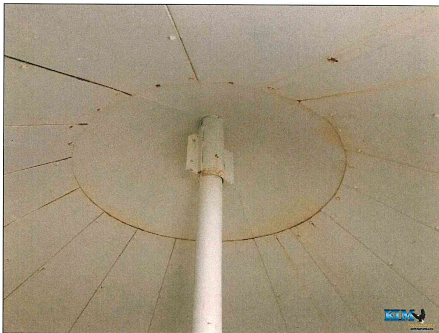
Photo No. 2 Overall condition of the roof
