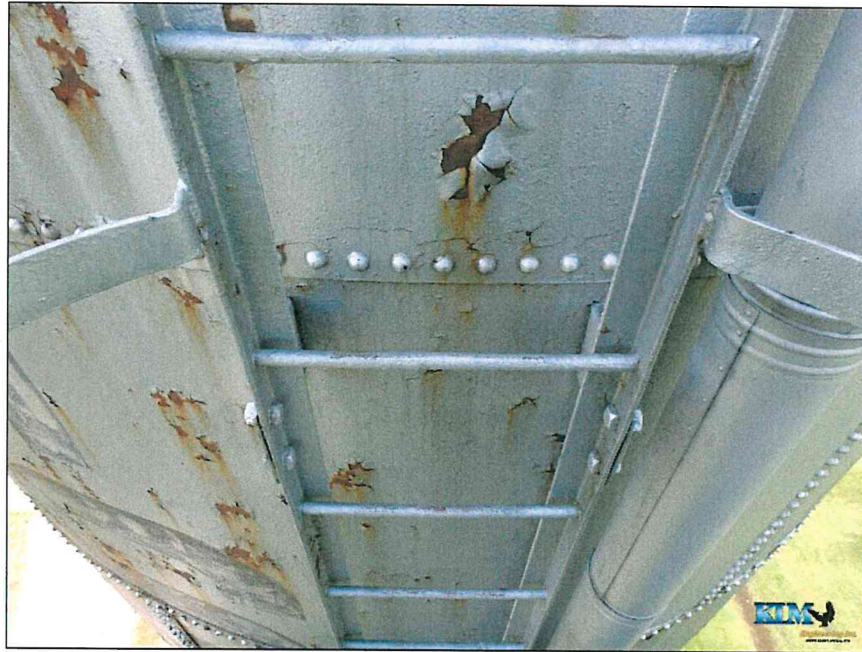
Photo No. 25 Condition of the upper shell and ladder
