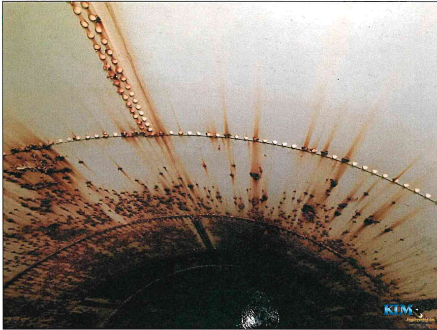
Photo No. 7 Condition of the upper shell courses
