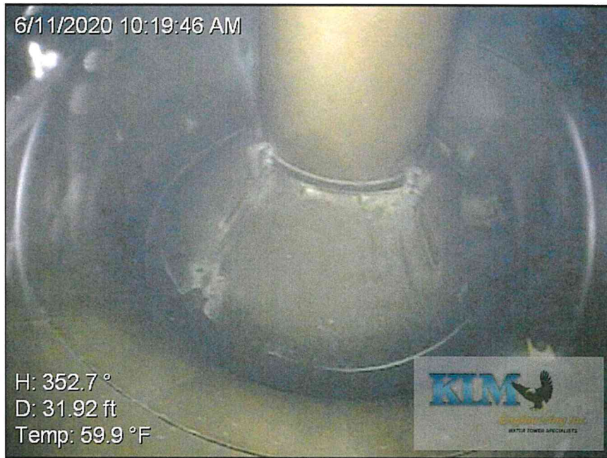
Photo No. 13 Overall view and condition of the bowl
