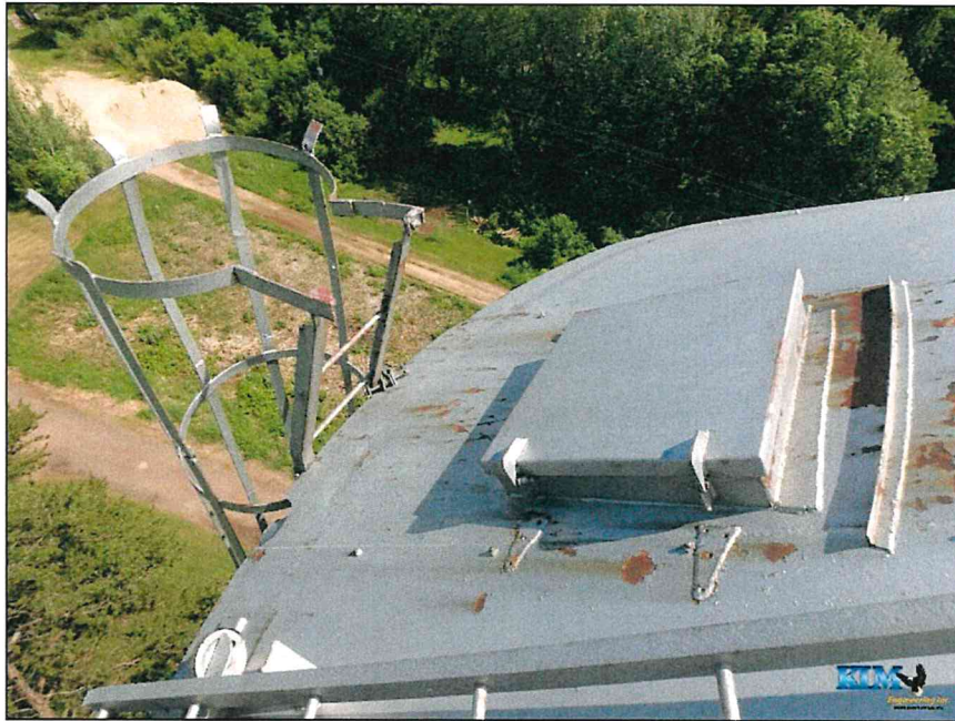
Photo No. 19 Condition of the roof, access ladders and access manway
