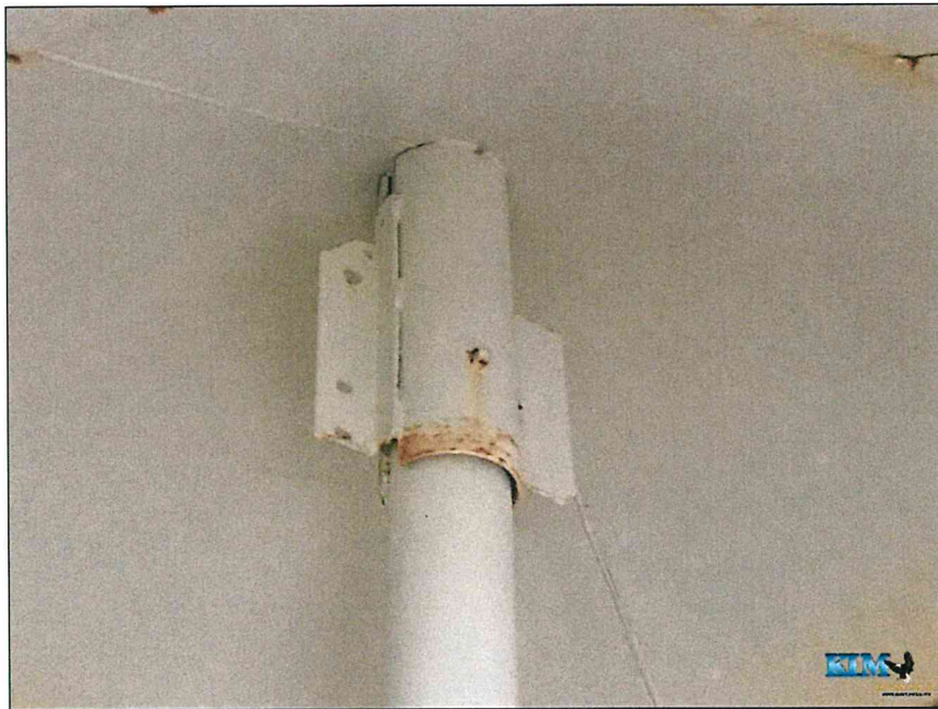
Photo No. 3 Center post at the top of the roof cone
