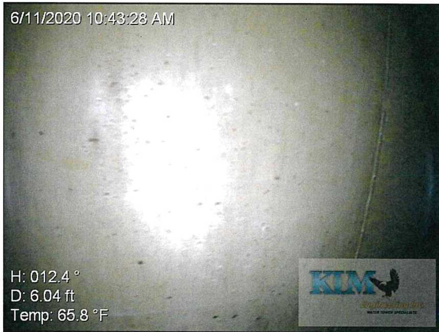
Photo No. 9 Condition of the shell below the water line
