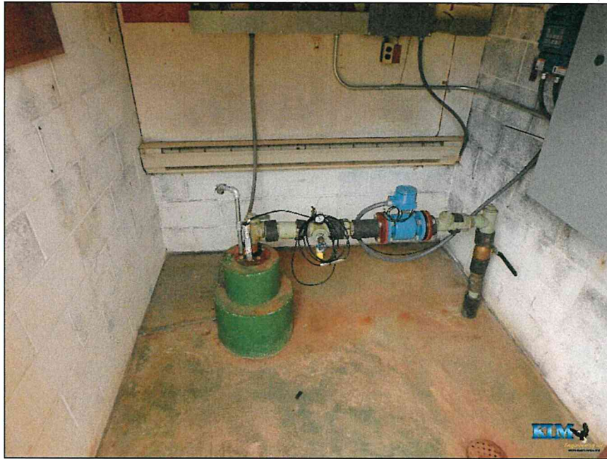
Photo No. 35 View inside the pump house
